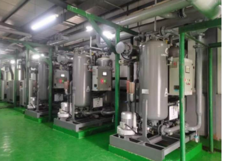
Project Client Chemical Industry Machine Model 6 × 32 m³/min Zero-Air-Loss Blower-Heated Regenerative Adsorption Dryers + Refrigerated Air Dryers
