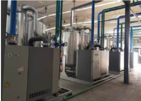
Project Client New Energy Industry Machine Model 3 Zero-Air-Loss Blower-Heated Regenerative Adsorption Dryers + 4 Stainless Steel Combined Air Dryers
