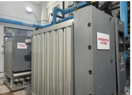
Project Client Power Plant Machine Model 2 × 75 m³/min Modular Adsorption Dryers
