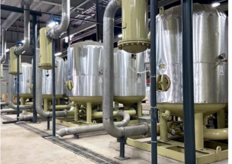
Project Client New Energy Industry Machine Model 12 × 220 m³/min Low-Purge Blower-Heated Regenerative Adsorption Dryers
