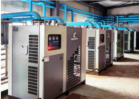
Project Client Cement Industry Machine Model 5 × 45 m³/min Refrigerated Air Dryers
