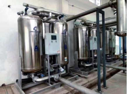
Project Client New Energy Industry Machine Model 8 × 95 m³/min Stainless Steel Adsorption Dryers
